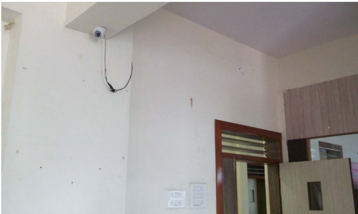
CCTV in the admin office
