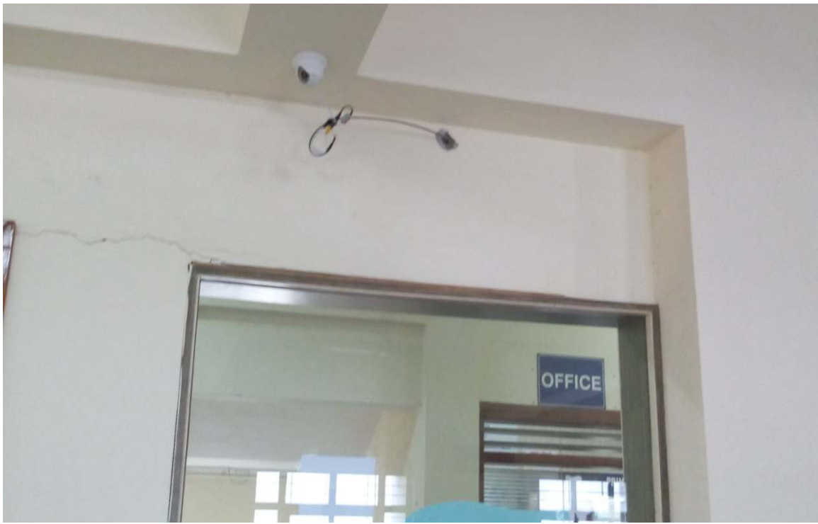
CCTV in the admin office
