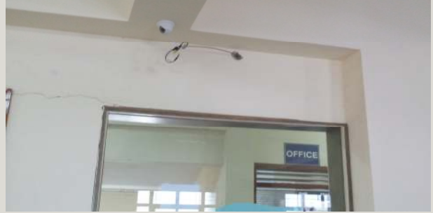
16 Additional CCTVs were installed at the institute
