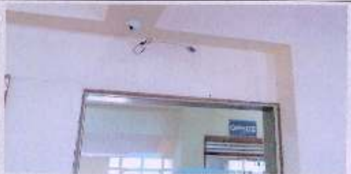
16 Additional CCTVs were installed at the institute
