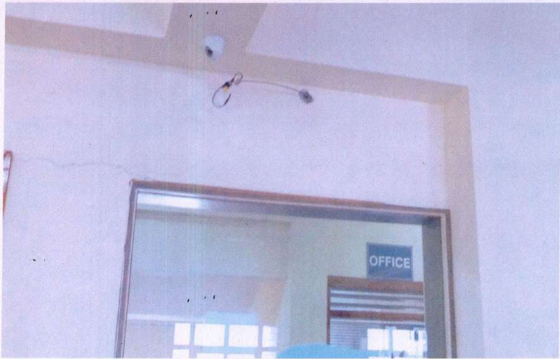
CCTV in the admin office
