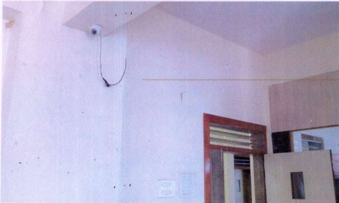
CCTV in the admin office
